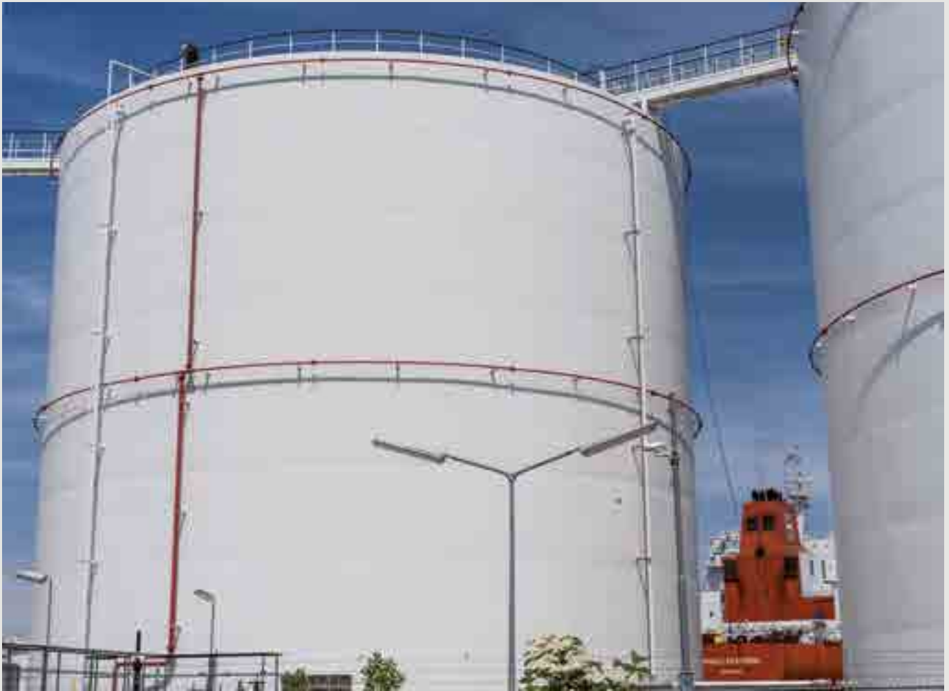
Around 50 percent of the fuels imported to West Africa come from Amsterdam, Rotterdam and Antwerp, collectively known as the “ARA” region. Port of Amsterdam, Netherlands, June 2016 | © Carl De Keyzer – Magnum
