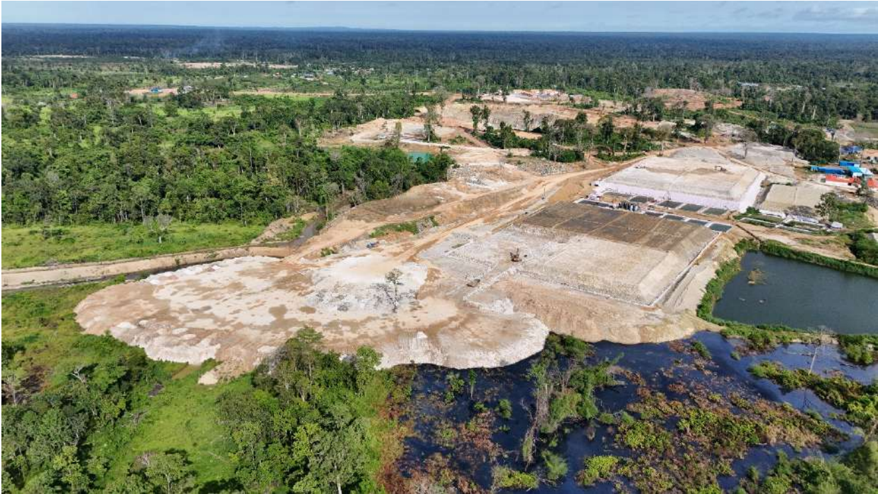
Figure 9b. (cont.). Drone imagery of Late Cheng main mine complex (Summer 2023).
