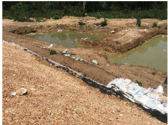
Probable cyanide leach field. Ponds in front of field.
