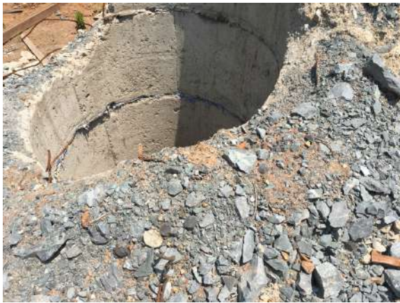
Gold Mining #5. Shaft with concrete casing.
