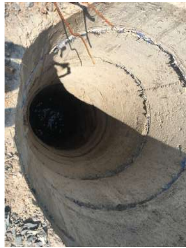
Gold Mining #5. Shaft with concrete casing.
