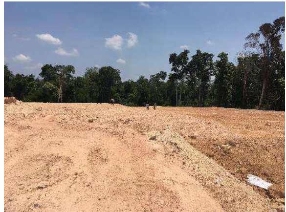
Probable cyanide leach field. Note people on top of field.
