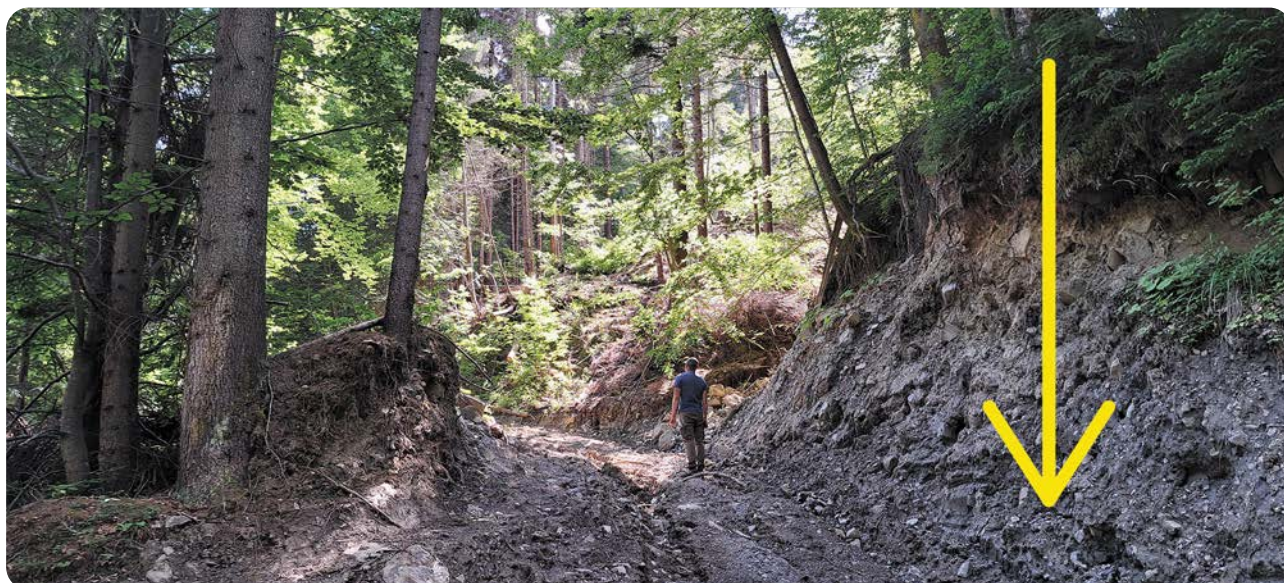
Soil erosion on the forest road in Ingka forest near Ceahlău, Neamț
