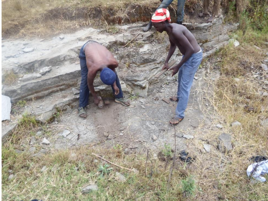
Picture 1: artisanal miners extracting pozzolana with chisels and hammers without wearing protective equipment. © TLC
